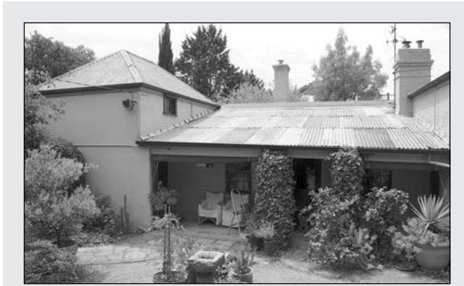
Graeme Davison, photographer Robert Hewett's house at Wesley Hill viewed from the side garden, 2014 The low slung central section, constructed with hand-made bricks, was probably the first to be built, but the original gable roof was later replaced with a skillion roof
