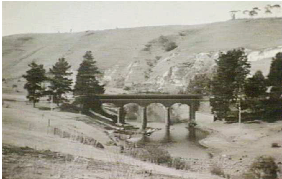
A view of Bulla Bridge over the Deep Creek near Greenvale, Vic. This bridge is one of blue stone & was built by convicts Date of creation: [ca. 1914-ca. 1941] postcard : printed, b&w ; 8.8 x 13.8 cm. approx. Reproduction rights owned by the State Library of Victoria Accession Number: H22840 Image Number: a08920 Collection: A.C. Dreier postcard collection
