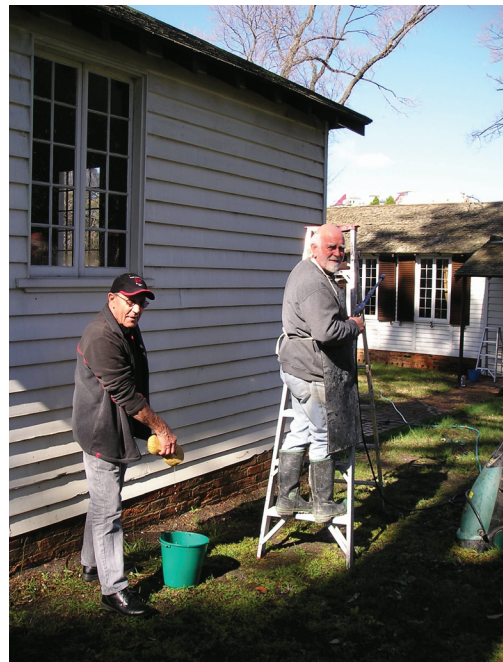
Peter Corlett and John Drury wash down the servants' quarters
