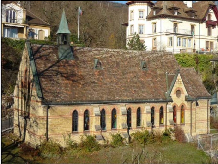
Raymond Berthoud, photographer La Chapelle de l'Ermitage, south facade, 2015
