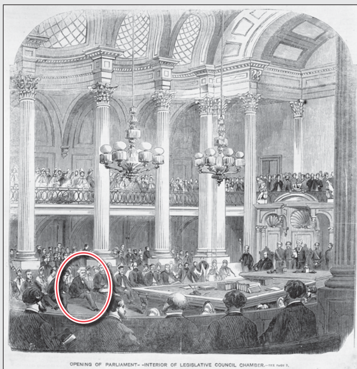
Samuel Calvert, 1828-1913, engraver Opening of Parliament — interior of Legislative Council chamber, 1864 Wood engraving Pictures Collection, State Library Victoria, IMP25/02/64/1 Published in The Illustrated Melbourne Post, 25 February, 1864 Captain Cole circled
