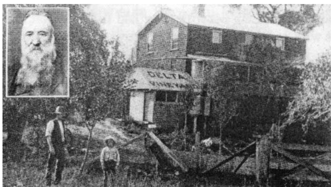
Professor Louis Wullemin's home, 'The Delta' Valencia Creek Road. The remains of this historic building can be seen on the west side of the Freestone just over the Delta Bridge. Inset: Prof. Louis Wullemin Discovering Briagolong
