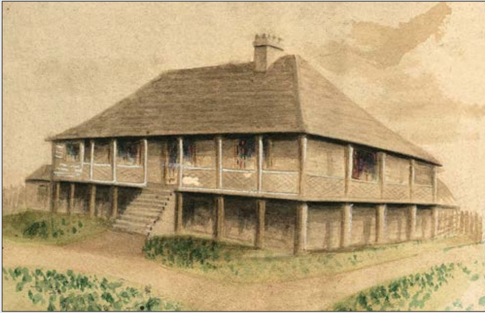
Aphrasia Cottage, Newtown, Geelong, 1853 Inset from Plan of Aphrasia Cottage & Grounds, Newtown, late residence of P.W. Welsh Esq. Geelong Heritage Centre Archives, 2030/A44 Plan signed by surveyor Joseph Shaw, 24 March 1853
