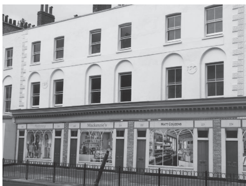
Figure 7 Benjamin Walmsley's former premises in London Road, London. Although now known as Nos 218-223, rondels at each end of the first floor level still indicate the original numbering of 126 to 128. Photograph: Simon Reeves, 2008.
