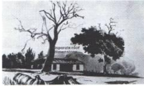
Fig. 3a George O'Brien (attrib.) Lonsdale's Cottage , c. 1850, with the disparate roof slopes marked, La Trobe Pictures Collection, State Library of Victoria, H3847.
