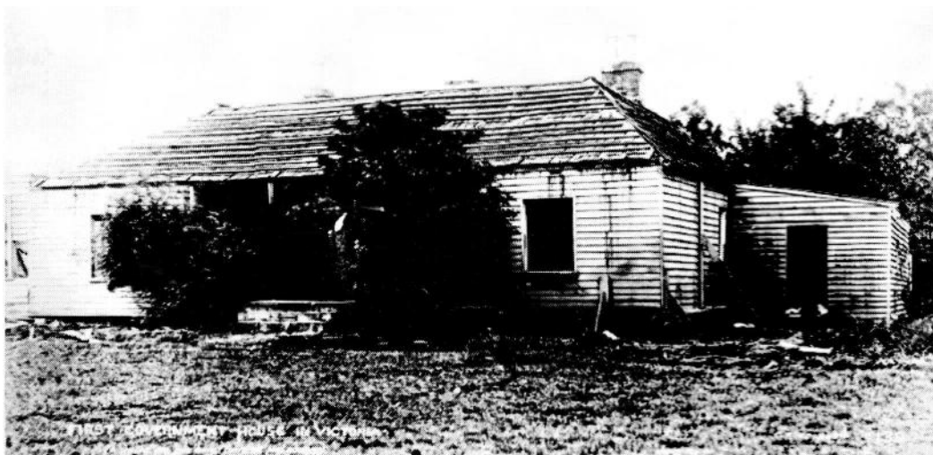
Fig. 6 Charles Rudd, First Government House in Victoria ; a relic of the early days of Melbourne - Lonsdale's Cottage, prepared for removal, 1891, photograph, La Trobe Pictures Collection, State Library of Victoria, H25802.
