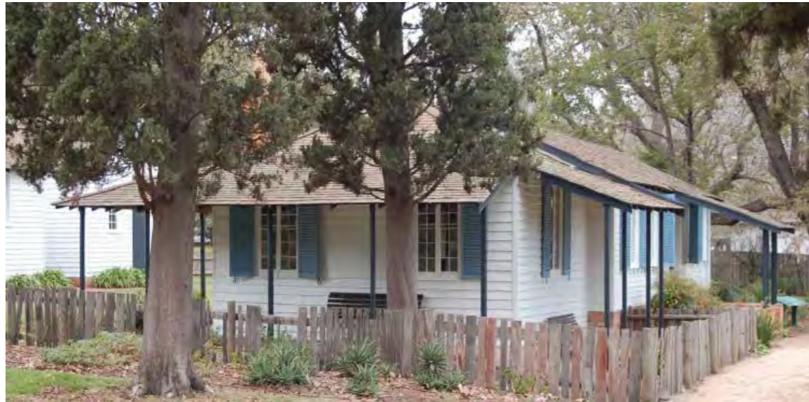
The newly painted blue shutters gleam on La Trobe's Cottage. This work was part of a package funded by a $60,000.00 grant from the Federal Stimulus package given to the National Trust. The blue colour was reinstated based on Gilbert's illustration. Other works included replacement of rotted timber, general external painting and reinstatement of part of La Trobe's dowelled picket fence.
