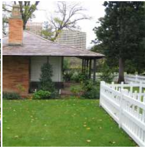
View down along the side of the Dining Room
