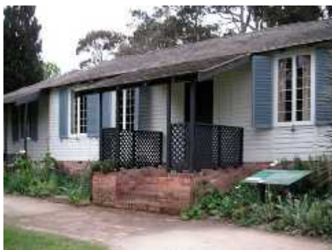
The cottage with its new lattice
